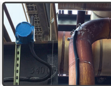
smartPIMS® Cellular with 3 dual-element sensors installed on overhead line.
